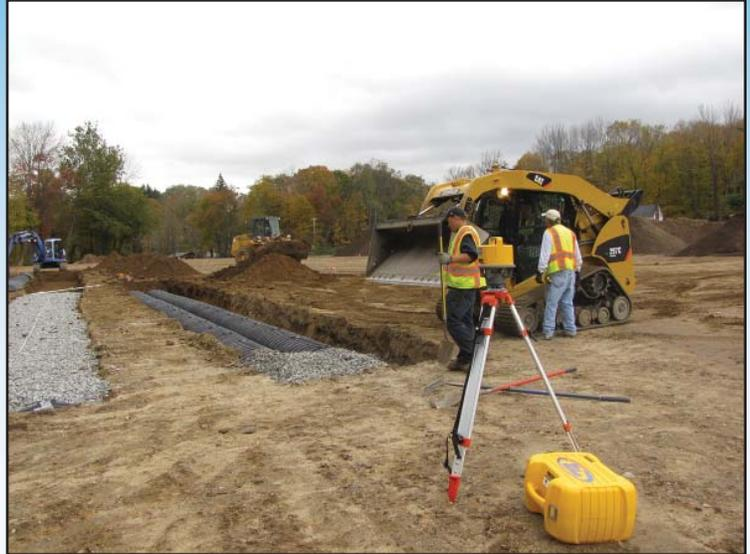
surface drainage of the soccer field and to provide nitrogen dilution. All of the chambers were placed on native material, and processed stone was placed above and on the sides of the chambers and topped off with common fill and topsoil.
