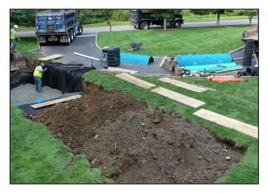
Recently, a high-end residence in Westport, CT had an existing competitor stormwater system that was not working properly. The system was not taking on water, and was completely silted. The home is located on a sprawling piece of property with beautiful green grass and a long asphalt driveway. The lawn and driveway were being destroyed by water collecting at the site due to the clogged stormwater system.
