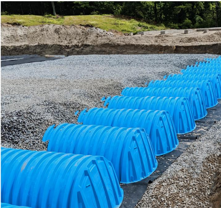
The CSA B184 standard covers polymeric subsurface stormwater management structures and accessories used in the collection, detention, retention, and infiltration of stormwater runoff. Applications include, but are not limited to, commercial, municipal, residential, agricultural, industrial, recreational, and highway drainage.
