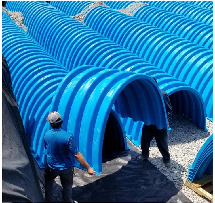
The CULTEC Recharger® Subsurface Stormwater Management System can be utilized in three ways as described in its NSAI Certificate, namely an infiltration soakaway, an impermeable attenuation system or a permeable attenuation system which combines infiltration and attenuation.
