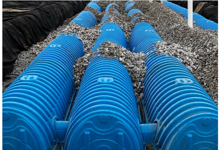
Several CULTEC Recharger® Subsurface Stormwater Chambers recently underwent this rigorous 3<sup>rd</sup> party testing – specifically the 150XLHD, 330XLHD, and 902HD chambers. All three chambers were found to comply with the standards set forth by the requested ETA, proving that the quality of the chambers stands up to project standards.
