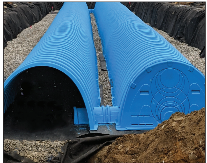
Shown: CULTEC HVLV FC-48 Feed Connector inserted into side portals of CULTEC chamber.
