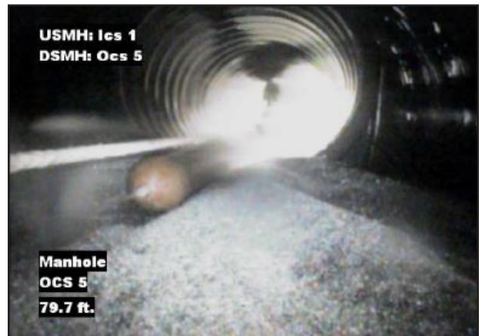
Cleaning ADS Isolator Row PLUS and pipes with high pressure water nozzle
