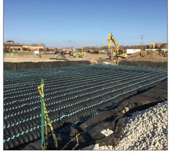
developments or redevelopments over the entire site for permeability. Since the soil at the site consisted of clay, the area to be developed cannot meet this infiltration requirement naturally and the project team was required to find a stormwater management solution that could allow for adequate storage until filtration could occur. Because of the limited green space of the area, the team found they would need to explore an underground chamber system.
