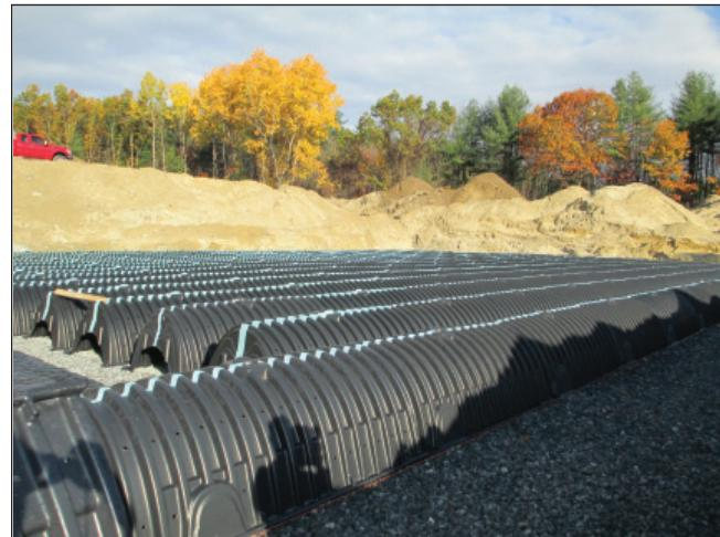
As of May 2015, two of the three stormwater fields are in the ground and backfilled and the foundation for the new assisted living facility is complete. The rest of the improvements are expected to finish in 2015.
