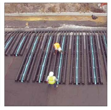
installed in an area where the water table is high, two different-sized chamber detention systems were used. The water is stored underground beneath the playing fields within the CULTEC systems until it is discharged downstream at a controlled rate.
