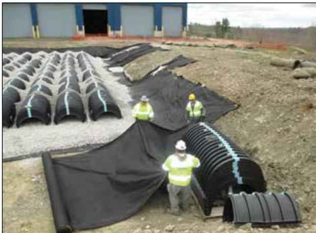
The CULTEC subsurface chambers work in conjunction with nine stormwater basins, catch basins, manholes and HDPE and concrete pipe to provide retention to the new site. Approximately 44% of total suspended solids are removed prior to the stormwater being directed into the CULTEC units, which then eliminate 80% of suspended solids via infiltration.
