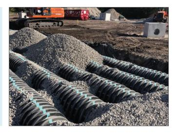
to switch from initial plans to use concrete materials to CULTEC's plastic chambers. The switch saved an estimated \$500,000 for Wawa's owners. The plastic chambers also allowed for more flexibility in the design and saved substantial time.
