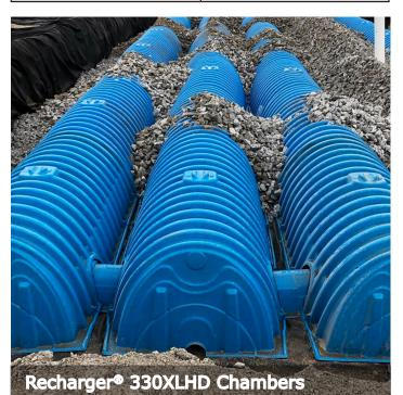
The first system is located under a grassy area and the second and third systems are beneath a parking lot for the wellness facility. The team chose to keep the systems separate because of differences in the water quality and volume. Since parking lot runoff is generally more contaminated than roof runoff to begin with, this water requires additional pre-treatment before entering the chamber system.
