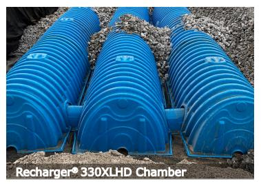
The team faced various challenges during the design and installation of the stormwater management system. Originally nicknamed the "Great Swamp" by early settlers in the 1700s, the site required prep work including site stabilization and purging as well as consideration of the site's high groundwater.
