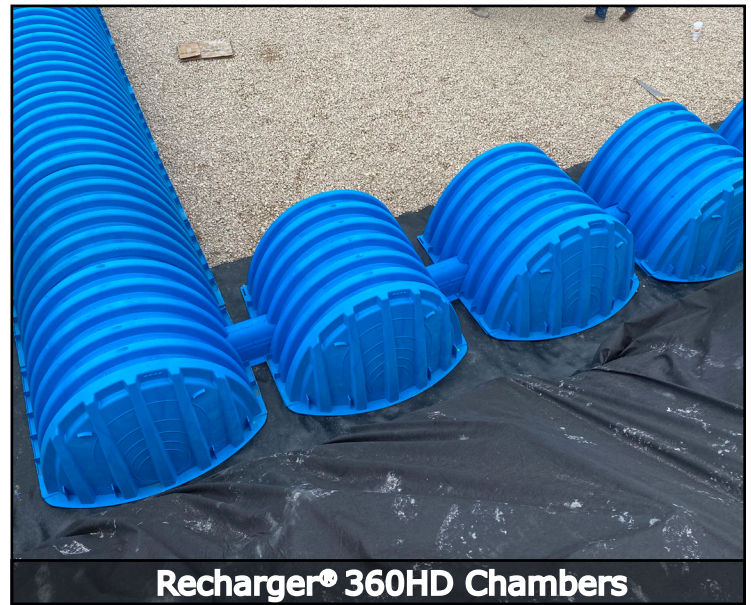
Figure 1: Stormwater Chamber Installation
