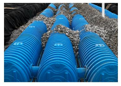
Several CULTEC Recharger<sup>®</sup> Subsurface Stormwater Chambers recently underwent this rigorous 3<sup>rd</sup> party testing – specifically the 150XLHD, 330XLHD, and 902HD chambers. All three chambers were found to comply with the standards set forth by the requested ETA, proving that the quality of the chambers stands up to project standards.
