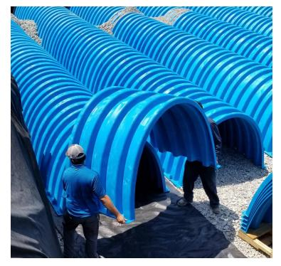
The CULTEC Recharger<sup>®</sup> Subsurface Stormwater Management System can be utilized in three ways as described in its NSAI Certificate, namely an infiltration soakaway, an impermeable attenuation system or a permeable attenuation system which combines infiltration and attenuation.
