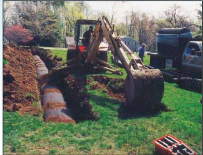
Trench installation demonstrating minimal disturbance of land.
